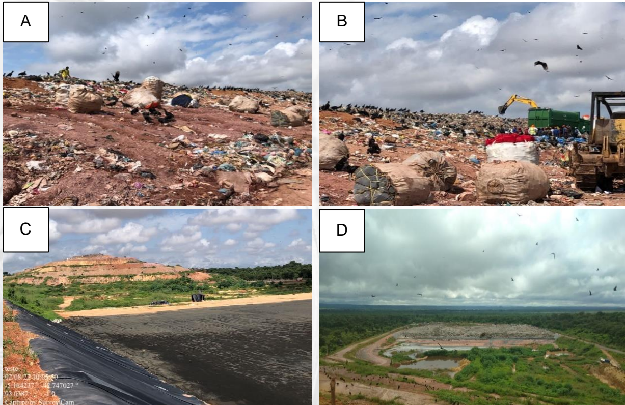
A. Waste pile in Cell 1; B. Machines working in the Cell 1 waste pile; C. landfill under construction (Cell 2); D. Cell 2 area with waste.
