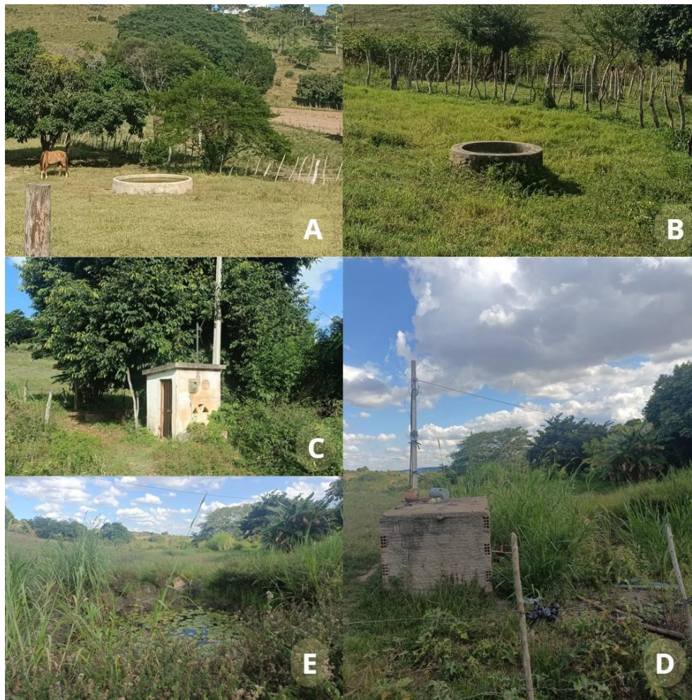
Figure 09 – Water Resources in the Region: (A) and (B) Amazonas wells; (C) and (D) drilled wells for groundwater extraction; and (E) a reservoir used for surface water storage.
